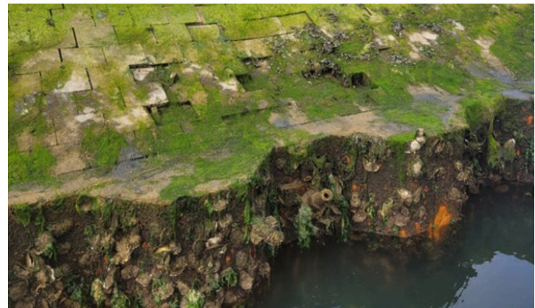
Dam wall with microbial corrosion.
